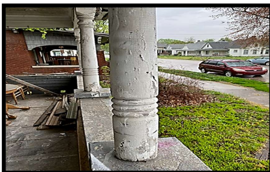
Lead covered porch column and windowsill
