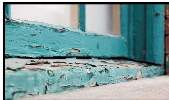
Lead covered porch column and windowsill
